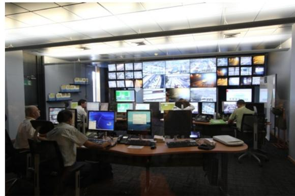
*Our student group visited a modern traffic surveillance center, shown here. CCTV cameras are used to monitor hazardous situations and dispatch police or road crews. Similar remote sensing, command and control tools can be used in a mining context.*
